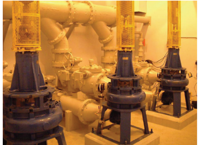
Figure 41. Sewage Pumps Mounted on Fabricated Stands.
